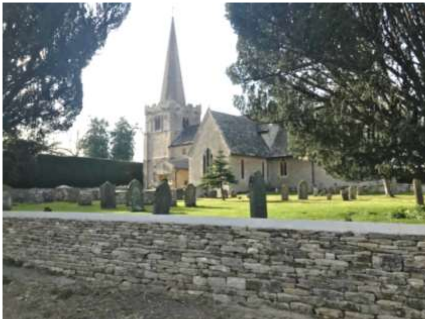
Image 1 - Drystone wall in the foreground is now restored.
