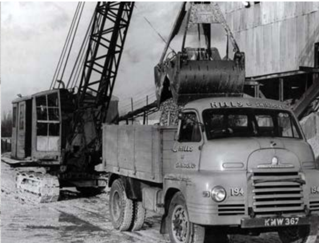
A Ruston Bucyrus excavator with grab loading an S-type petrol Bedford six-tonne tipper at the Broadway Lane North Gravel Plant, South Cerney.
