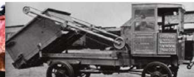
An early brick delivery lorry. This four-wheel drive vehicle had a mechanical container for tipping its entire load.
