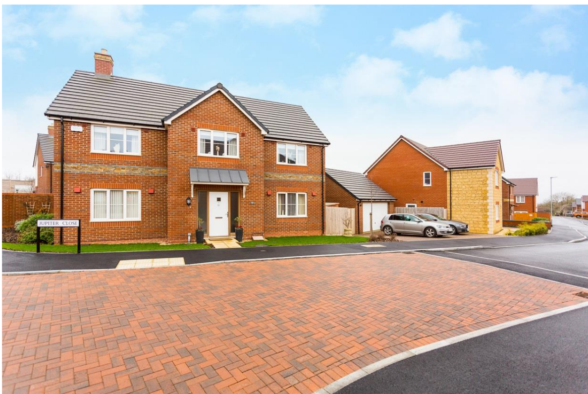
Hills' development, Hillside, Blunston, shortlisted for a West of England LABC Building Excellence Award.
