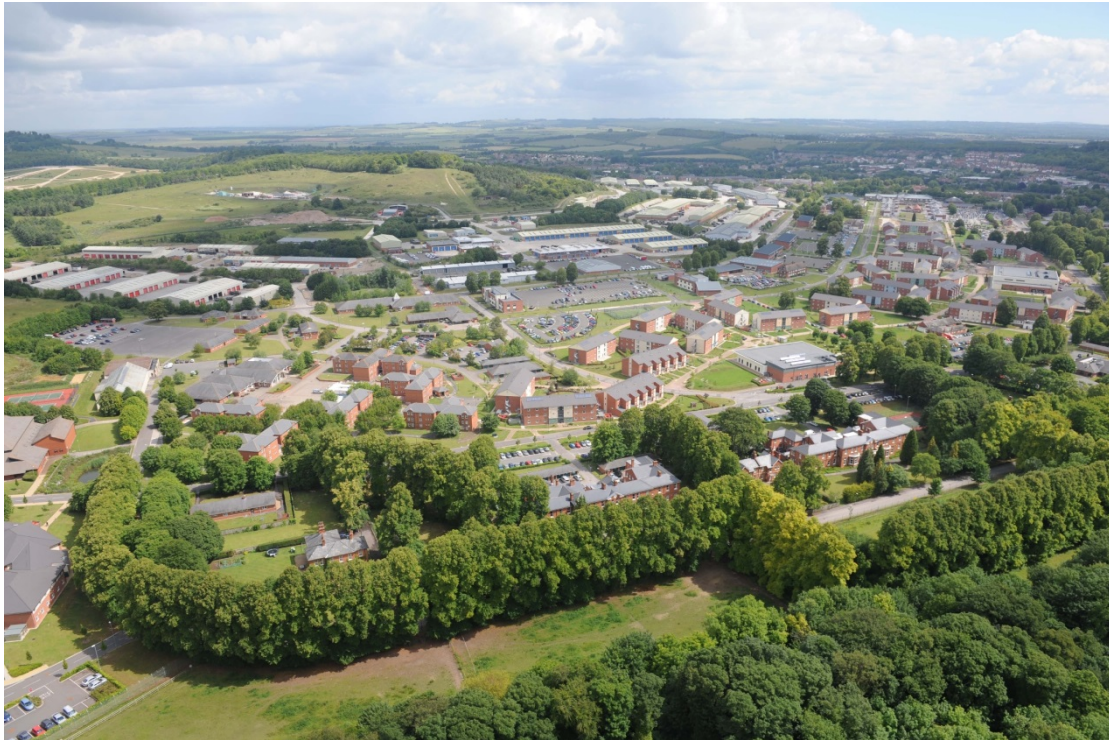
Aerial view of one of the PAC garrisons covered by the waste management contract
