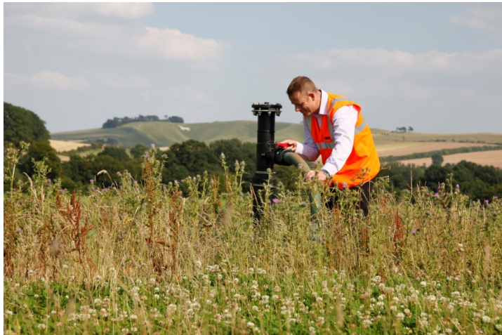
Image caption : Management of the gas extraction system on a restored landfill now used for agricultural activities
