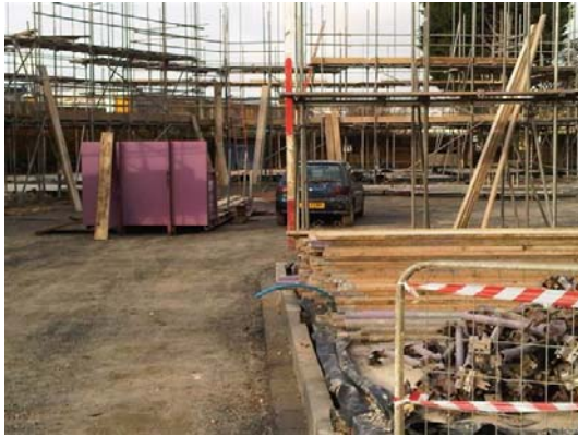
Jan 2012 – Construction begins
