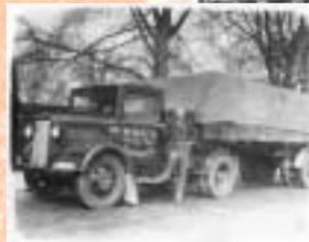
*An early brick delivery vehicle from the 1920s. This four-wheel drive lorry had a mechanised container for tipping its entire load*
