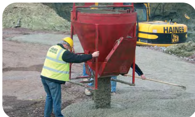
Ready-mixed concrete being poured from a skip and then raked into position
