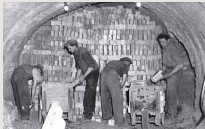
Stacking the continuous kiln at Purton
