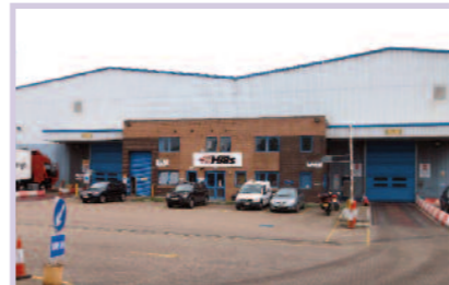
2013 The Amesbury Recyclables Management Facility opens after a five month fit out.
