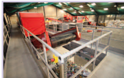
2012 Sorting equipment including an optical separator is installed at the Porte Marsh Recyclables Management Facility to process cardboard and plastic bottles.
