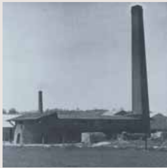
Chimneys at Purton
