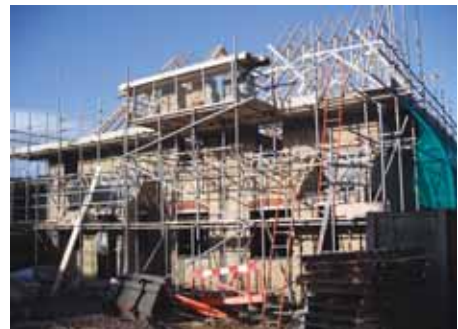
One of the houses under construction at Purton
